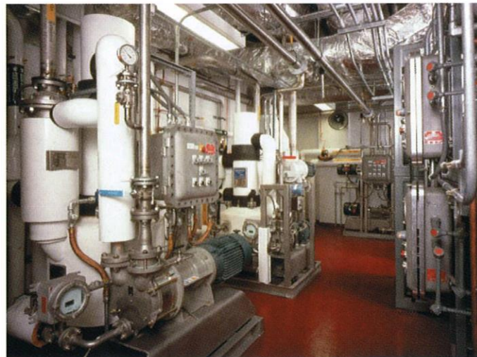
Figure 5. Temperature and vacuum control of the reactor systems is accomplished via vacuum and TCU skids located in the mechanical rooms.
