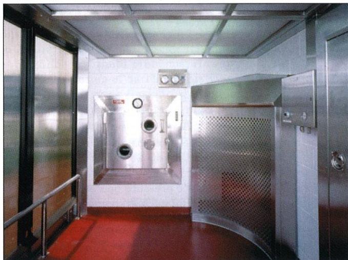
Figure 4. Curved exhaust manifolds complement the HEPA filtered downflow ceiling design.
